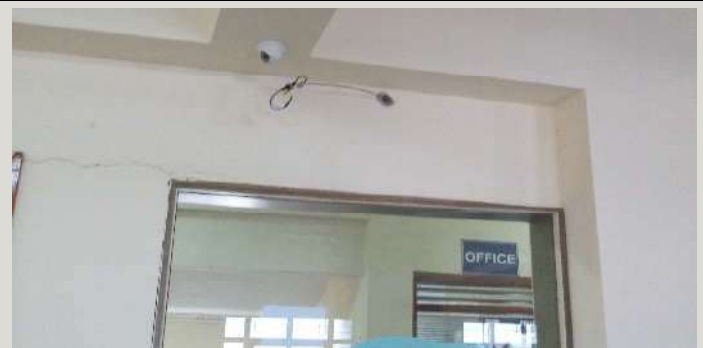
16 Additional CCTVs were installed at the institute
